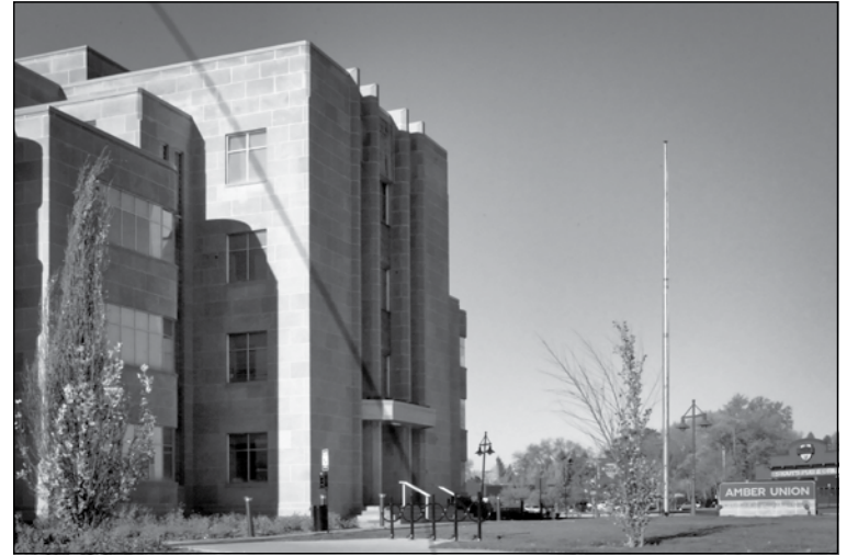
Developers of Amber Union (pictured above) are planning an addition to the site called Amber Flats. Photo by Lou Michaels.
