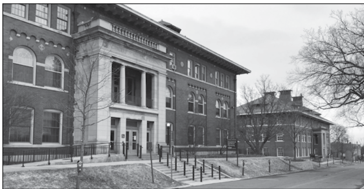
University campus buildings in St. Paul along Eckles. Photo by Kristin Anderson.
