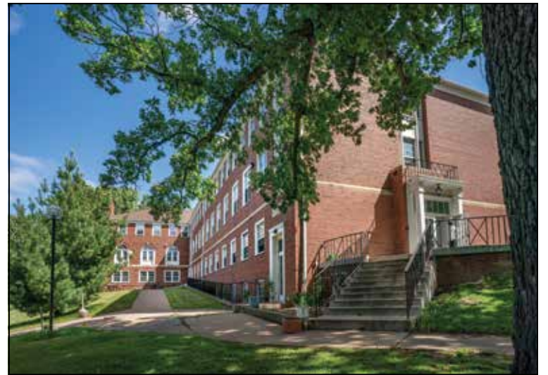
Luther Seminary's vacant Stub Hall was proposed to be used for a homeless shelter. The seminary canceled in the wake of neighborhood concerns. Photo by Courtney Perry, courtesy of Luther Seminary.
