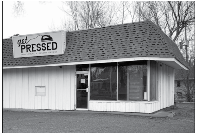
By one estimate, the bill for environmental clean-up of the long-vacant dry cleaners at Larpenteur Avenue and Albert Street could exceed $350,000. Photo by Bill Brady
